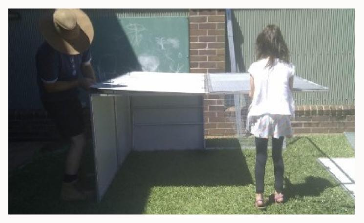
3. Get your assistant to lift the middle meshed panel to waist height. This will allow you to attach the back panel using 5 bolts. If you have a stronger helper than I, it is easier to attach the back panel with the roof door opened completely (180 degrees) and laid back on the mesh panel provided the assistant can hold the weight.
